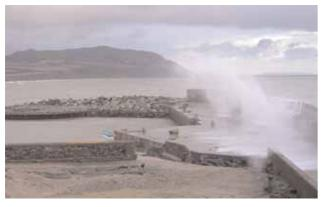
these and the slope absorb waves. The Sea Walls in Bangor, Co. Down are similarly designed. I have seen large waves hit it and appear to vanish into it.
