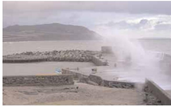
The wall has been designed for the higher sea levels expected with Global Warming. The height is a compromise between the need to preserve the sea view from the Public Square and stopping waves coming over. The curve on the sea side of the top of the wall throws back most of the waves which reach it.
